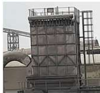
Coal Transfer point Bag filter
