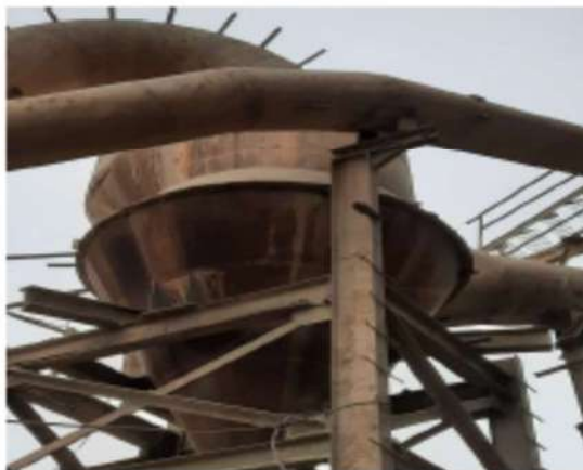
KF Bin hopper venting cyclone dust collector
