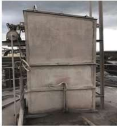
Fly Ash Silo De dusting Bag Filter
