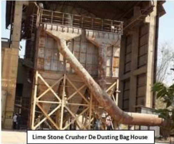
LS Crusher Transfer Point (BC4) Venting Bag Filter
