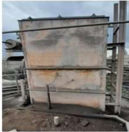
Bed Ash Silo Bag Filter
