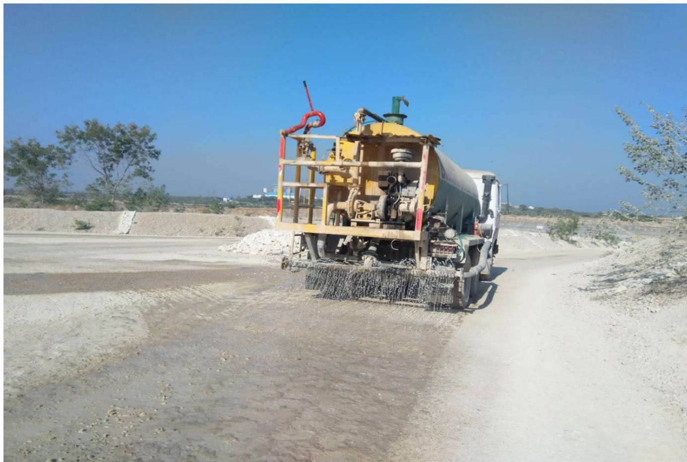
Haul Road wetting with water tanker
