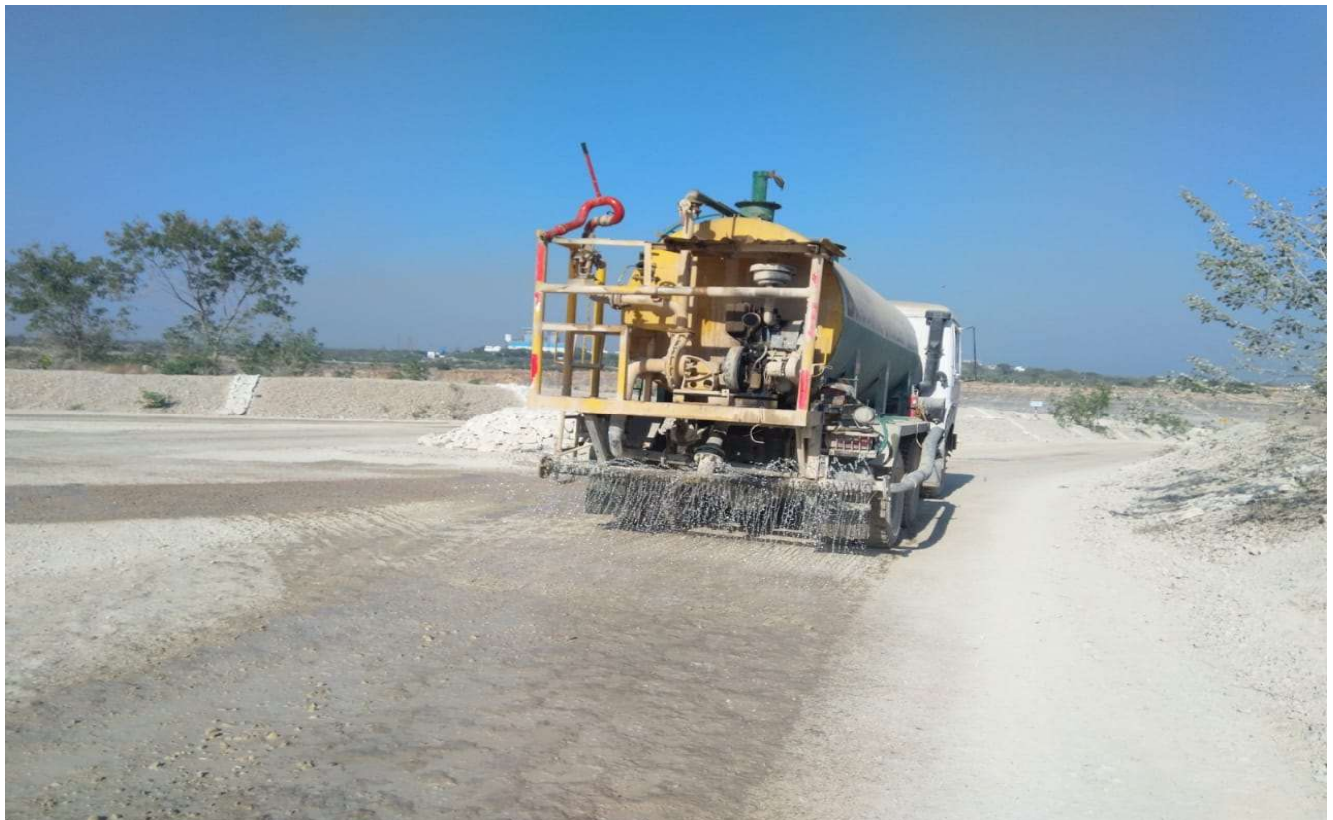
Water Sprinkling with Tanker for Dust Suppression.
