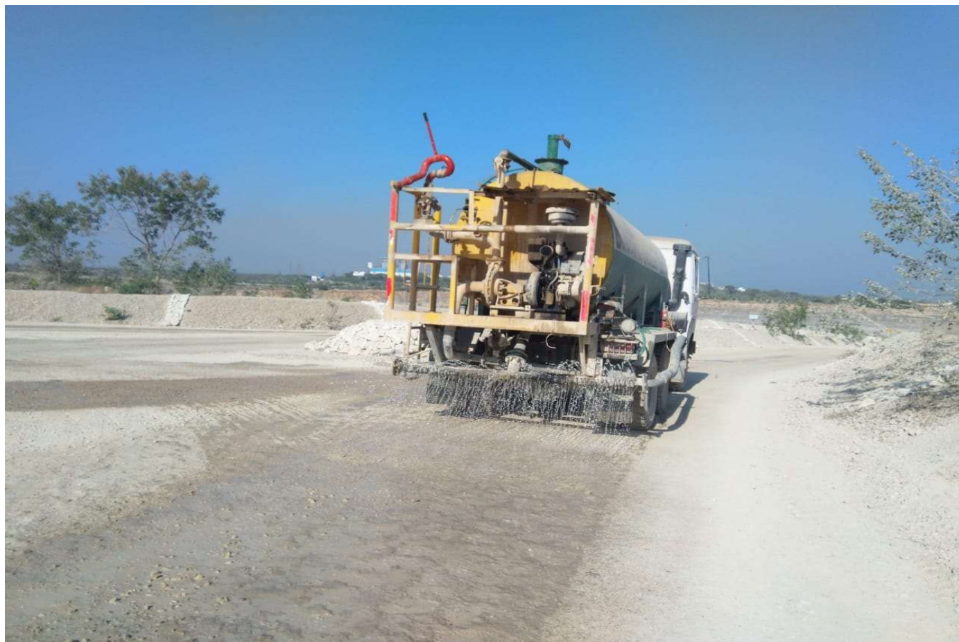
Haul Road wetting with water tanker
