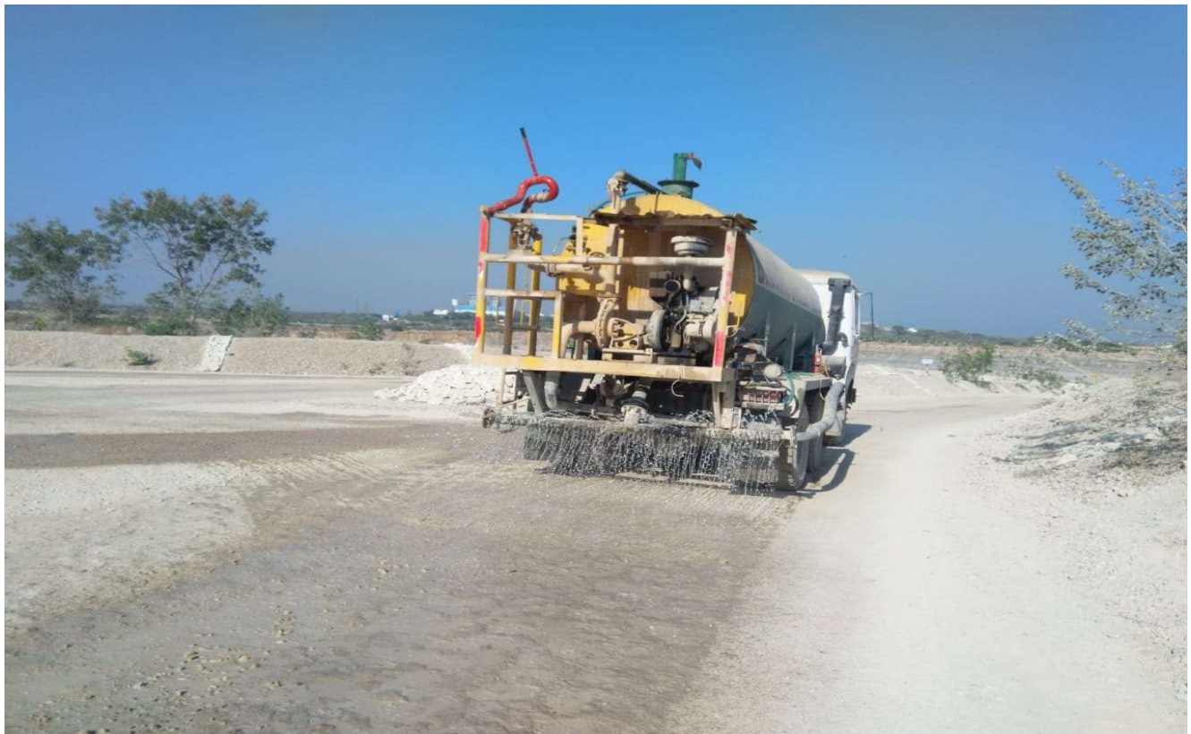
Water Sprinkling with Tanker for Dust Suppression.
