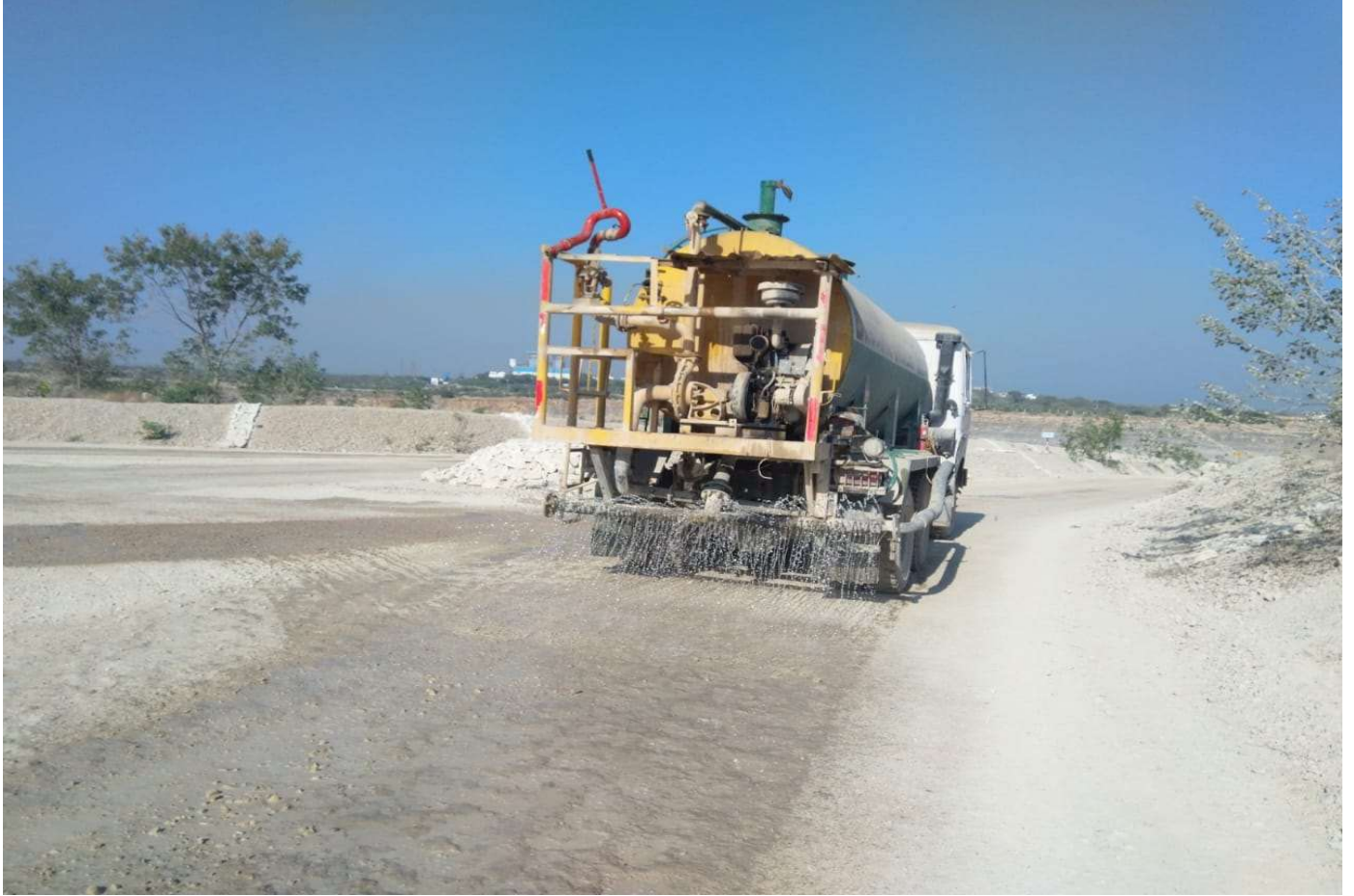
Haul Road wetting with water tanker
